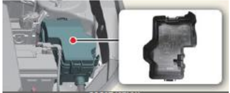
Engine room fuse box
